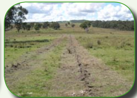
Figure 5. A site in the early stages of bed preparation, the first fallow knock-down spray is taking effect and the site has been deep ripped.
