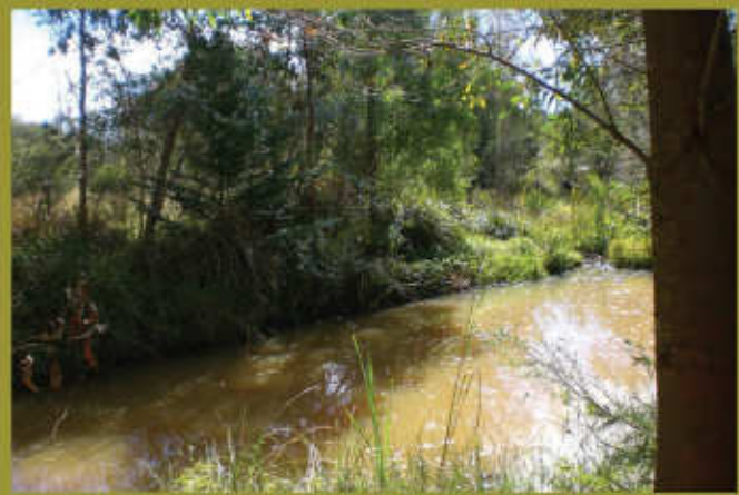
Figure 3 Maitland St., Rock Ramp Scheuberger After
