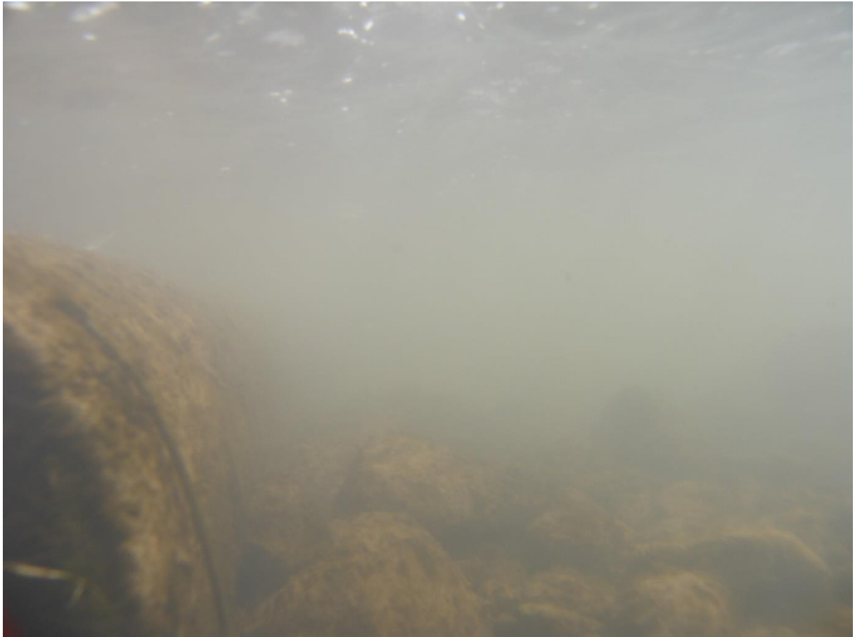
Figure 8. The logs were partially buried in the sediment and fencing wire was used to anchor the logs to the star pickets.
