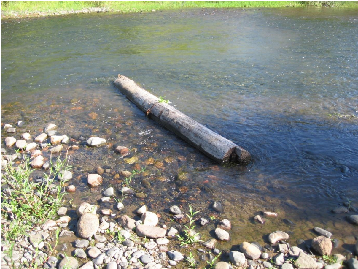
Figure 6. A close up of a log step comprising two 'fence-post' sized logs in the Hunter River downstream of Muswellbrook. Notches were cut into both ends for attachment to star pickets to anchor the step-jam in location. Accumulated fine sediments can be seen on the upstream side of the log. This photo was taken during very low flow conditions.
