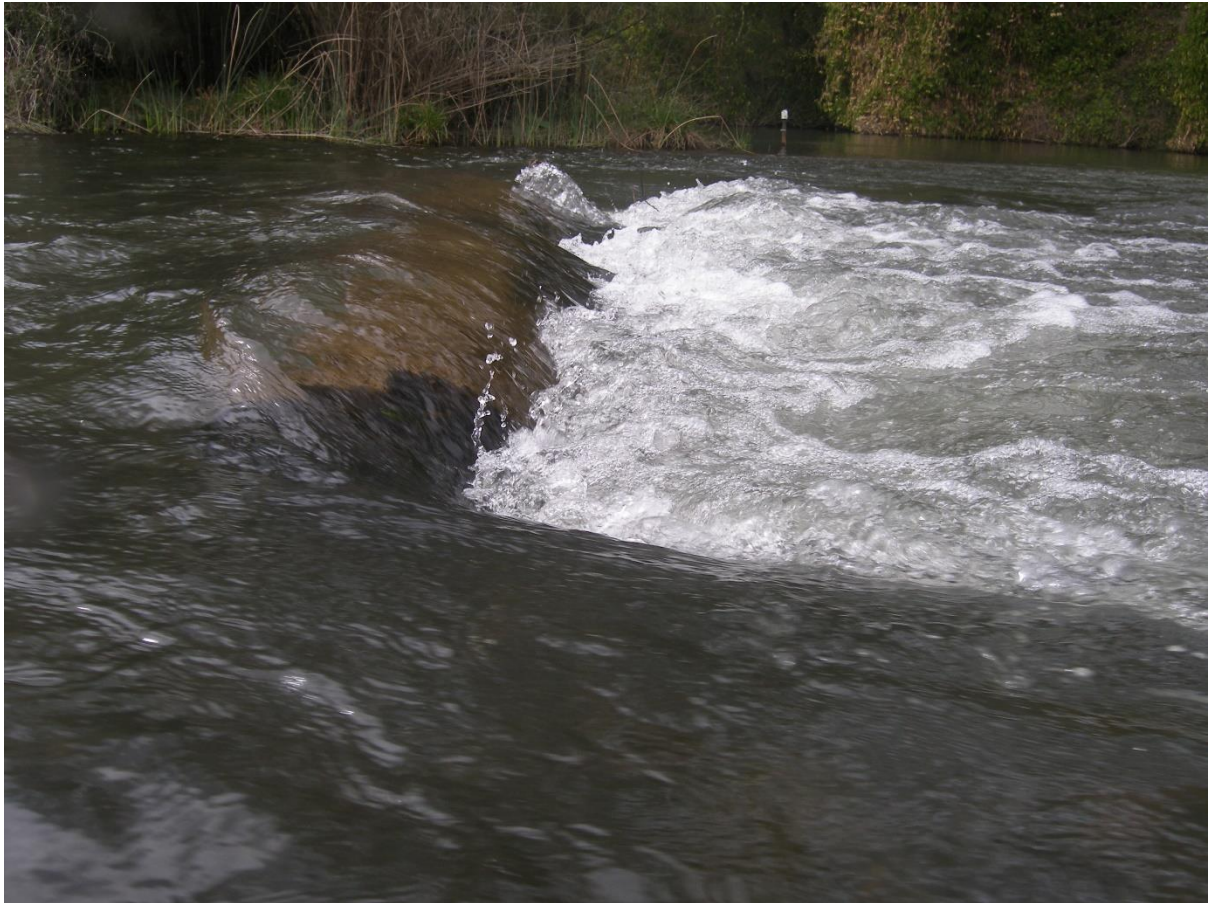
Figure 7. A similarly constructed log step-jam under high flows. The hydraulic jump and turbulent water are clearly visible. A small scour pool formed immediately downstream of the log from the turbulent flow, creating a small sediment dune immediately downstream of the pool. Sediment accumulated immediately upstream of the log, embedding it further into the stream bed. This created an area of complex topography and range of microhabitats in a previously homogeneous streambed.
